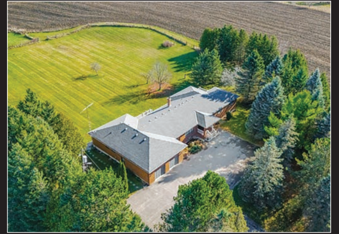
KING 52 acres in prime sought after location with custom built estate home!
