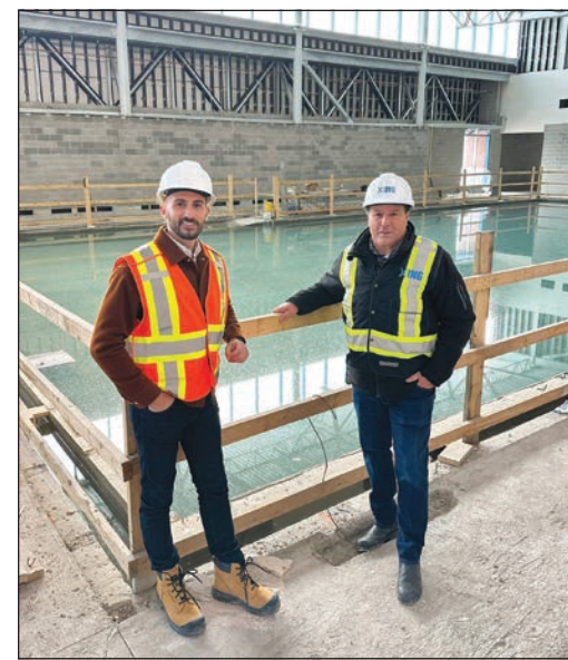
MPP Lecce tours the construction of the new Zancor Centre, with Mayor Pellegrini.
