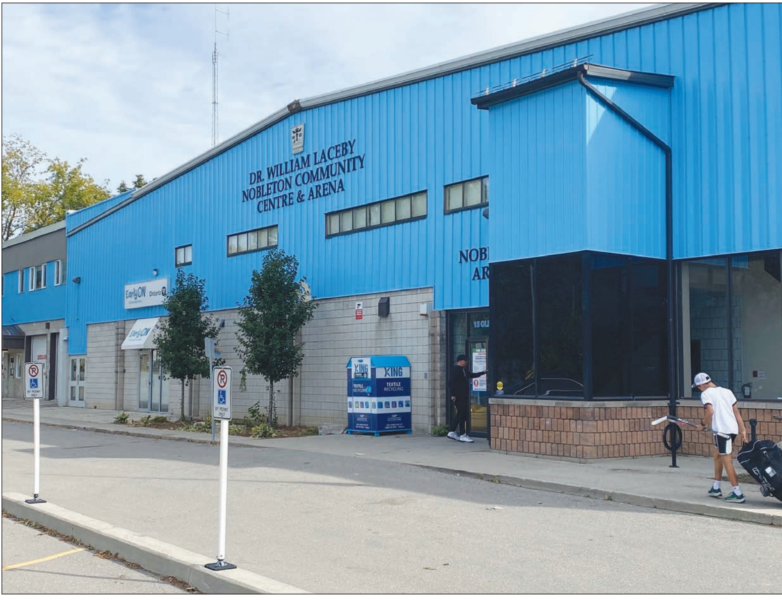
The Dr. William Lacey Nobleton Arena is closed pending urgent mechanical repairs.
