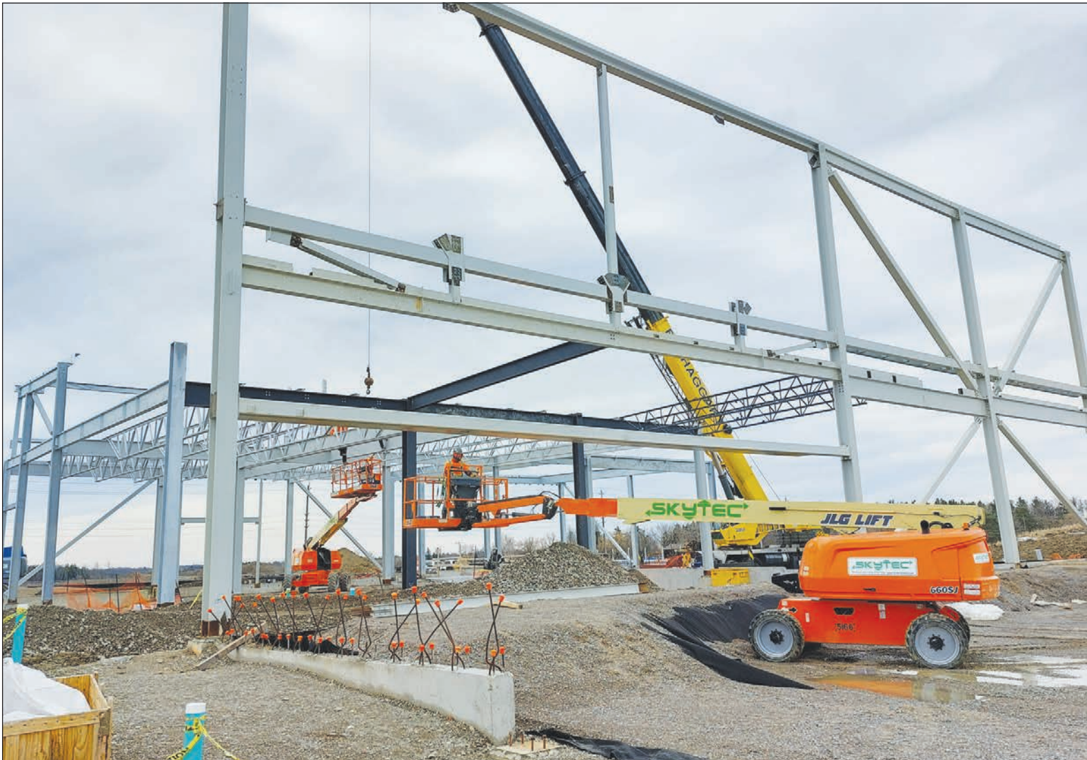
Work progressing on rec. centre
