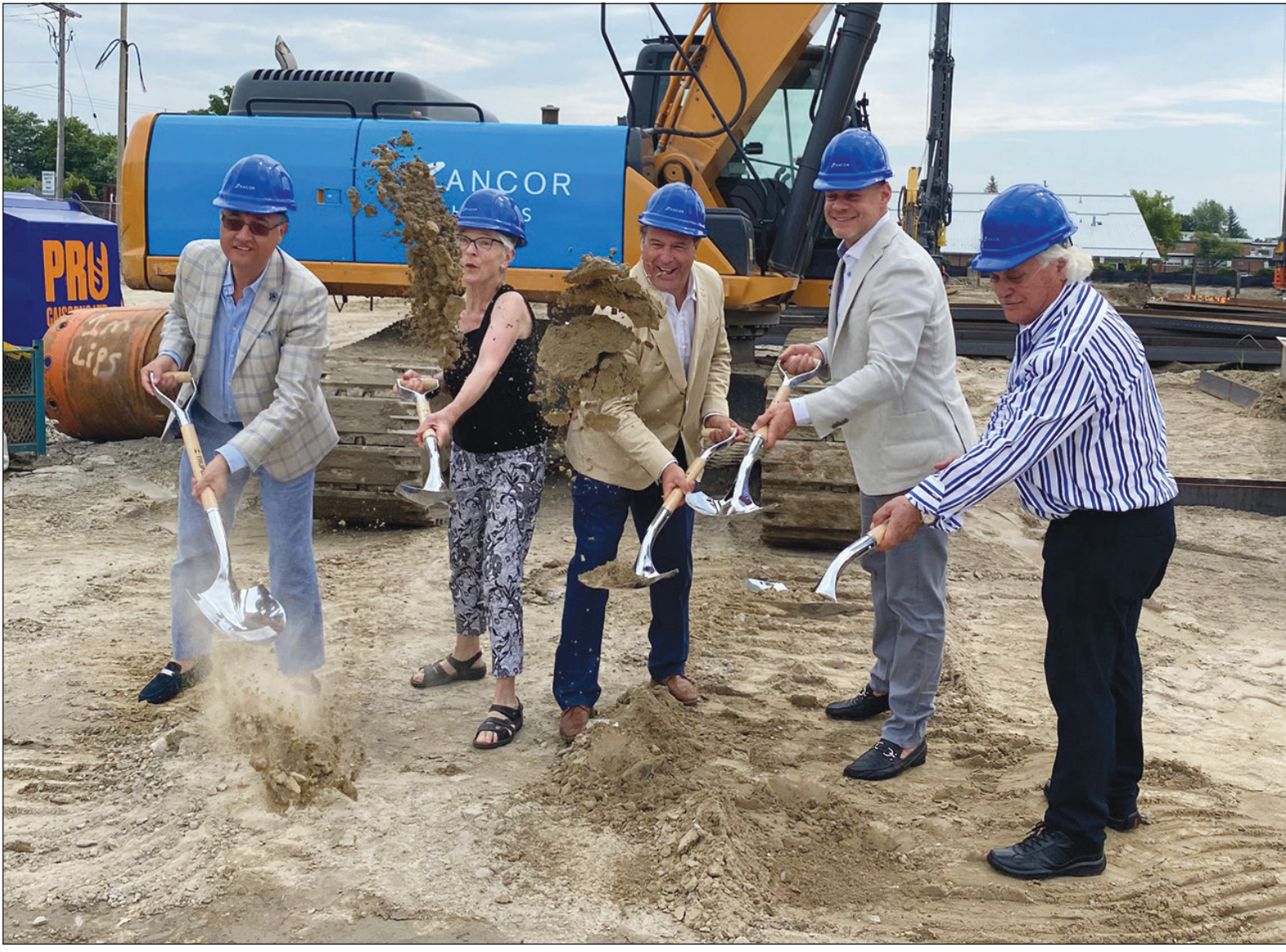
The shovels hit the ground for the ceremonial ground-breaking of King Terraces in King City, a 6-storey condo development by Zancor Homes. On hand for the ceremony were (l to r) Anthony Pignetti, Councillor Debbie Schaefer, Mayor Steve Pellegrini, Fabrizio Cortellucci and Nick Cortellucci.
