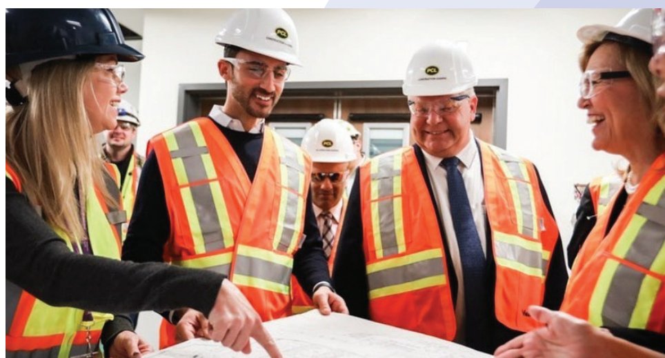
Stephen and Doug Ford touring Cortellucci Vaughan Hospital during the construction phase in 2019
