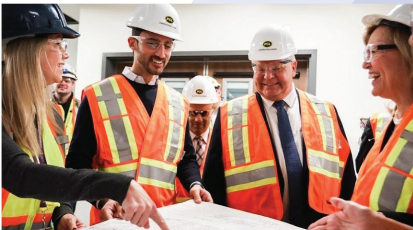
Stephen and Doug Ford touring Cortellucci Vaughan Hospital during the construction phase in 2019
