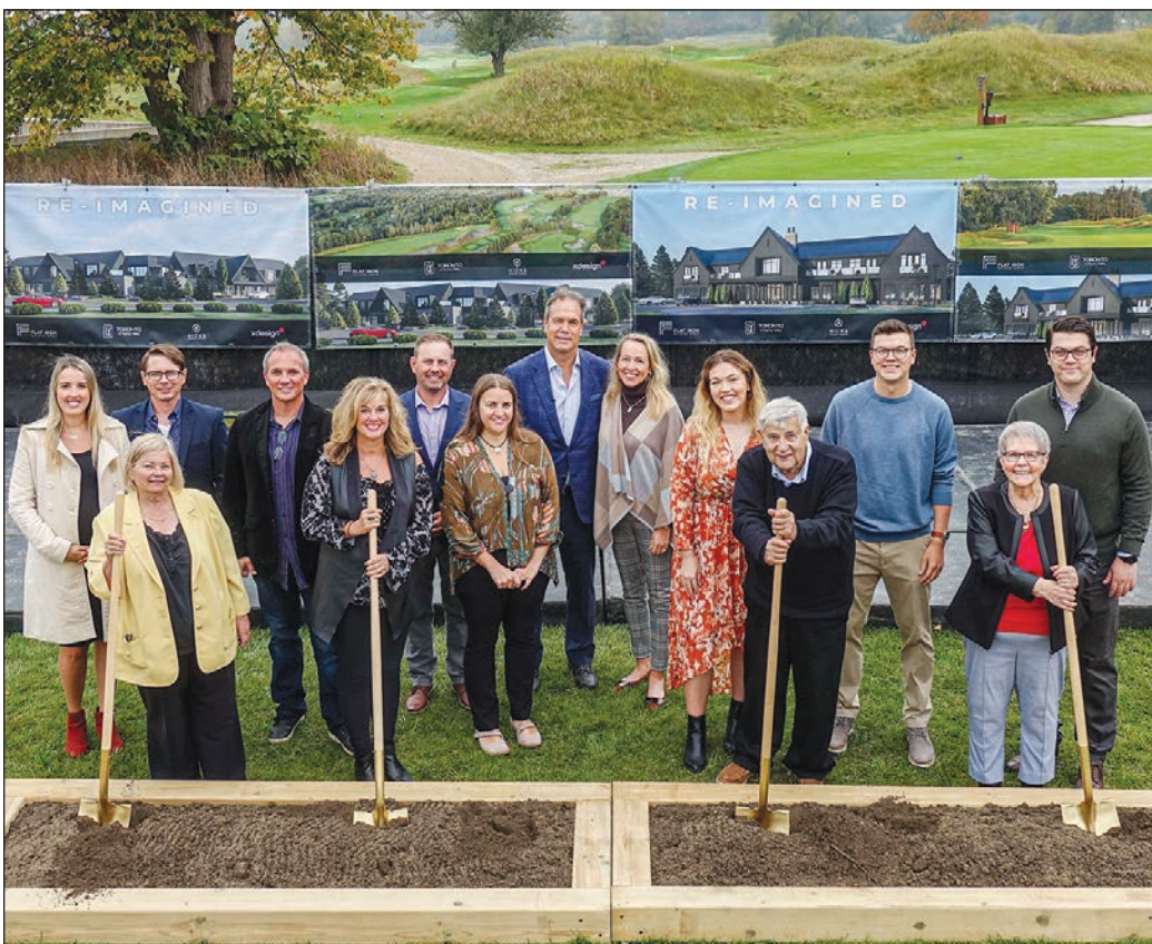
The Humeniuk family celebrates the ground-breaking of their new construction project that will consist of building two new clubhouses and more.
