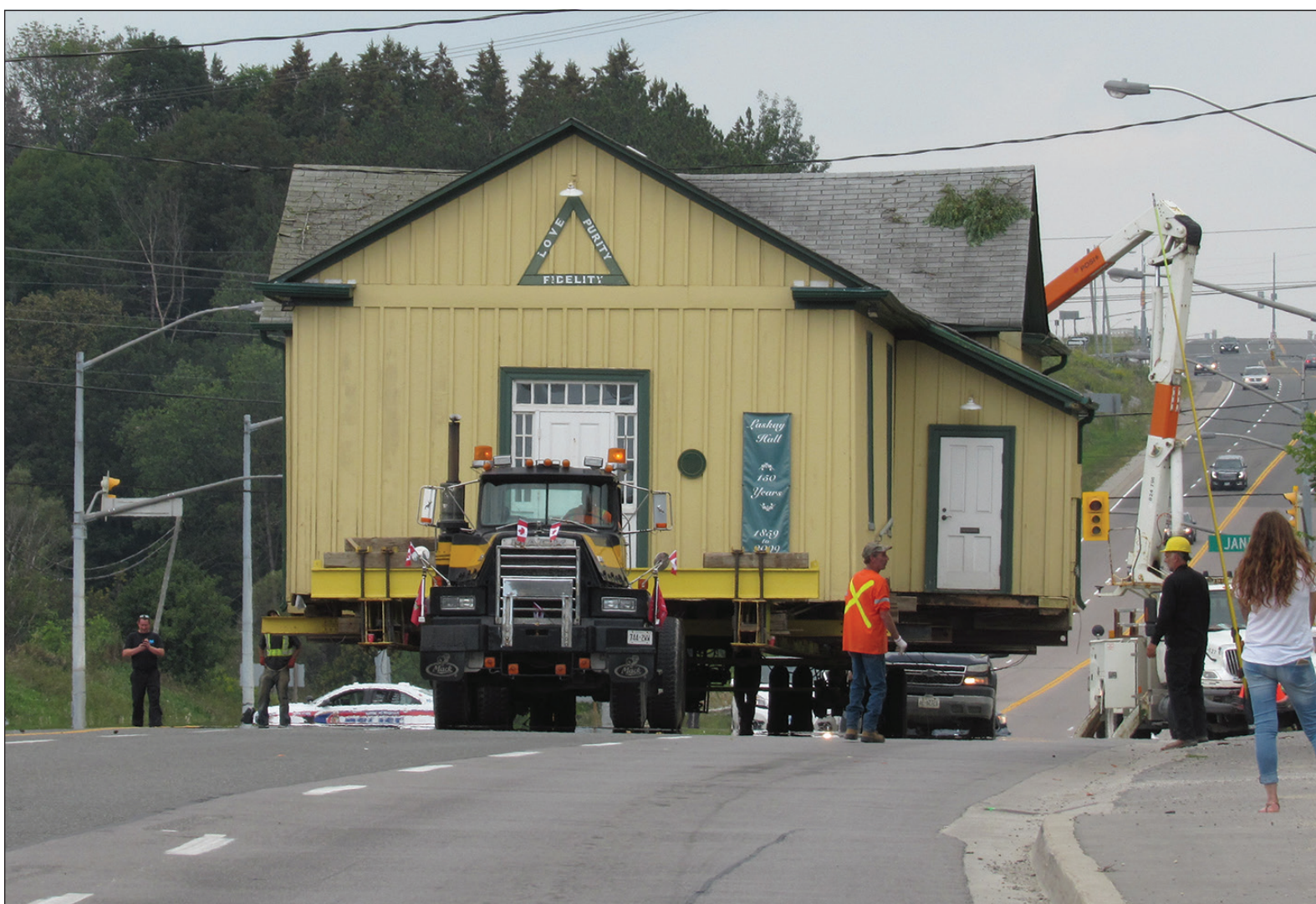
The historic Laskay Hall was picked up from its home on Weston Road, and carefully moved to its new home on King Road, at the King Cultural Centre last week. Moving at roughly 5 km/h, the hall made the trek, unscathed, in roughly four hours.
