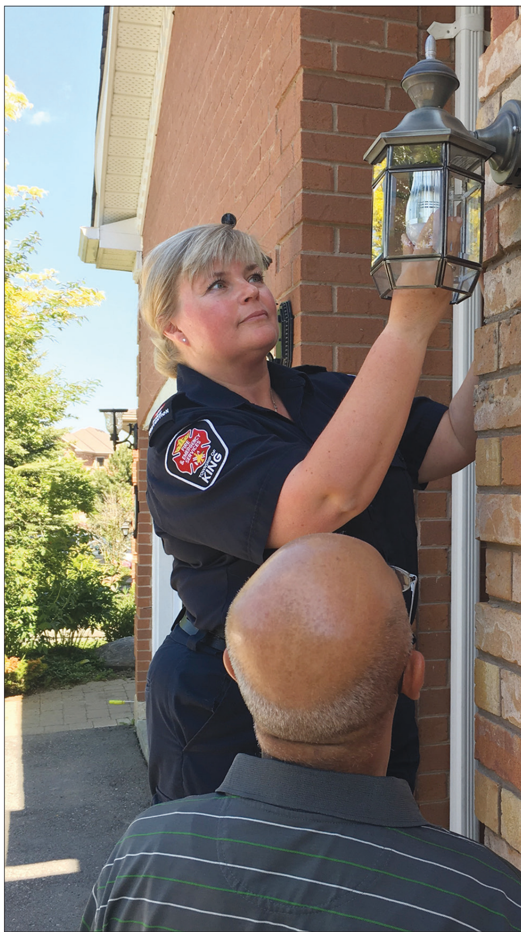
Shelley Langer, of King Fire & Emergency Services, installs a guide light at a local resident's home. This new campaign will make it easier for emergency personnel to locate the home of someone in distress.
