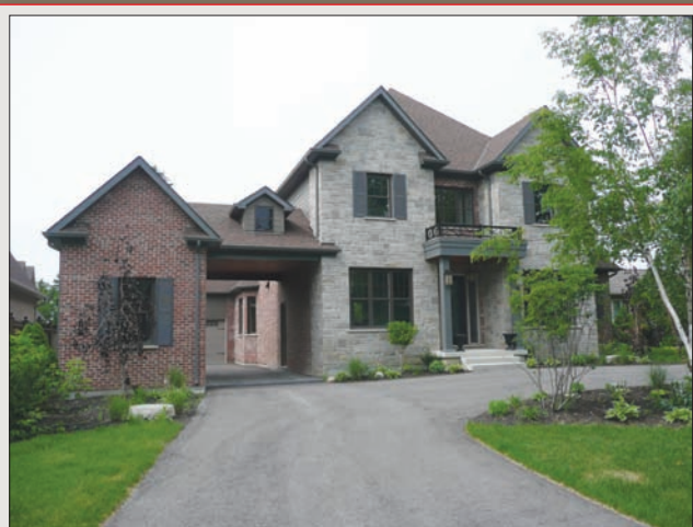
RICHMOND HILL NEW CUSTOM BUILT HOME! 75x200 FT. LOT, $1,888,000
