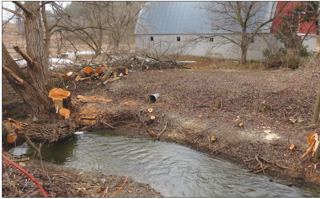
The bridge project by the Schomberg Community Farm is a go. It's been funded by the community, along with major sponsors that include King Township and Trisan Construction.
