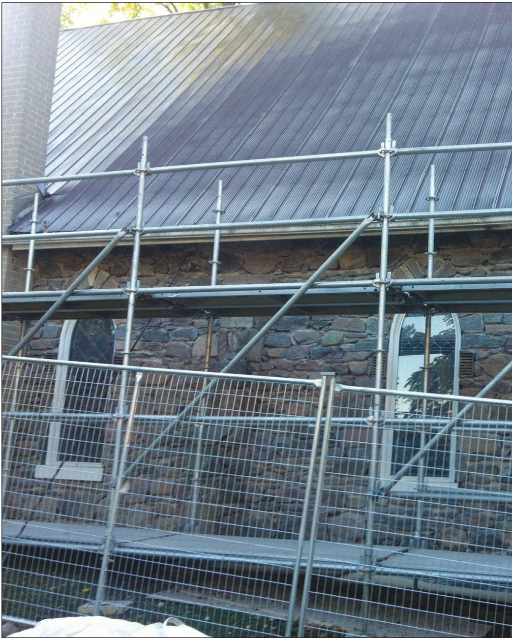
Work has begun on Kettleby's Christ Church roof restoration.
