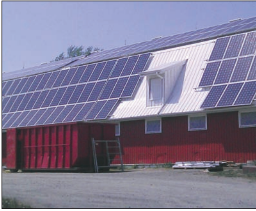
Kinghaven Farms currently boasts just over 1,000 solar panels on its barn rooftops, producing 265kW. They are applying for an additional 1.2 MW.
