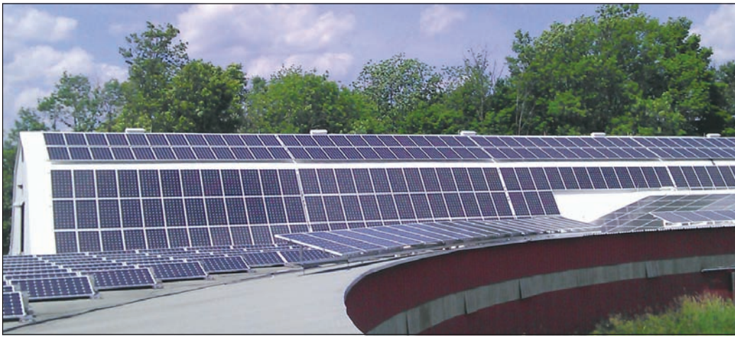
Kinghaven Farms currently boasts just over 1,000 solar panels on its barn rooftops, producing 265kW. They are applying for an additional 1.2 MW.
